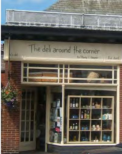
1930s detailing at 61 Hotspur Street
