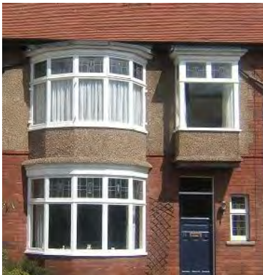
Roughcast render above brick on Queensway
