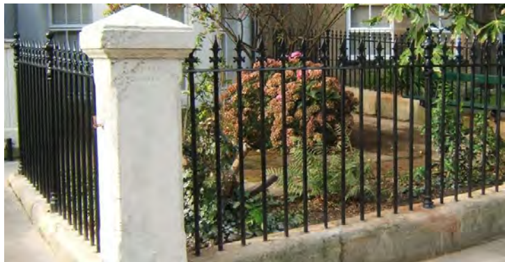
New railings in an accurate, traditional style at Priors Terrace
