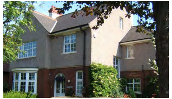
Gable at 18 Manor Road
