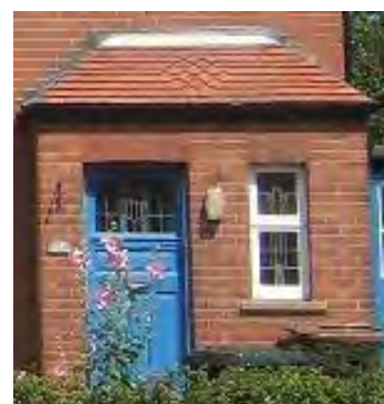
Brick porch on Queensway
