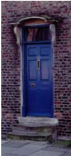
AN ATTRACTIVE DOORWAY FROM THE 1740S SET IN A WALL OF HANDMADE BRICKS. THE STONE HOOD IS TYPICAL OF THOSE ONCE FOUND ELSEWHERE IN THE CONSERVATION AREA.
