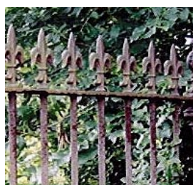
EXAMPLES OF ORIGINAL CAST IRON RAILINGS TO BE SEEN IN TYNEMOUTH.
